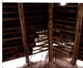
道均洋桥廊屋梁架 Beams of lounge house on Daojunyang Bridge
